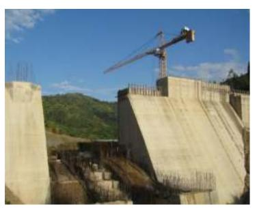
Another important aspect of mass concreting in dams is the use of formwork. Formwork is a temporary structure used to support the wet concrete until it sets and hardens. The formwork must be strong enough to support the weight of the concrete without collapsing or bending under the pressure. To achieve this, formwork is usually made of steel or timber and designed to withstand the weight of the wet concrete.
